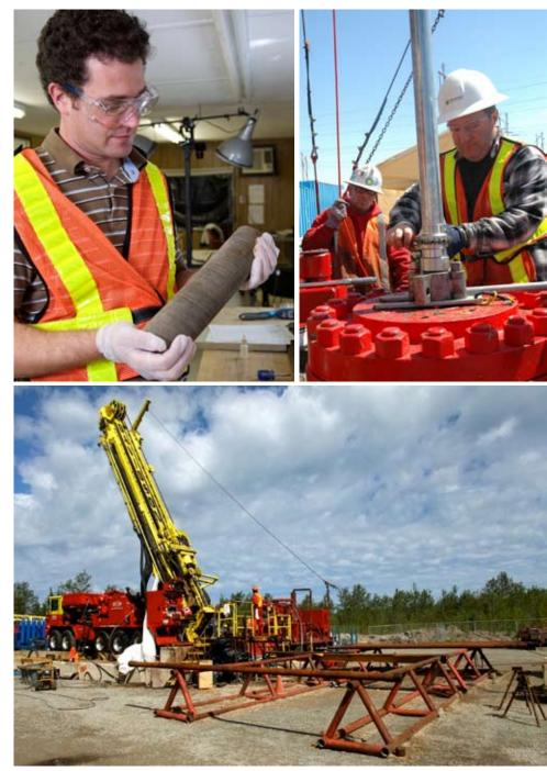
Top left: NWMO engineer Dylan Luhowy examining rock core Top right: Multi-level monitoring system installation Bottom: Inclined borehole drilling
